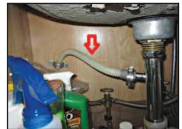
Drain Missing High Loop
